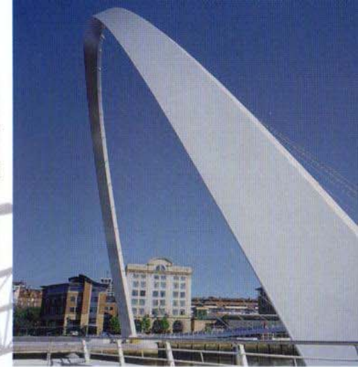
Image courtesy of Gateshead Council. Photograph: Doug Hall of 121
